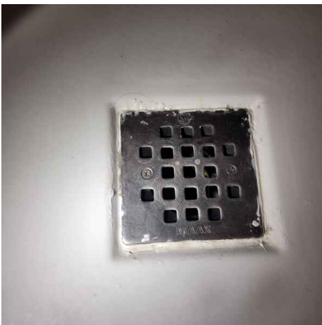
Remove cover and reinstall correctly
