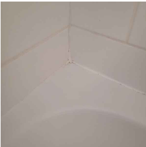
Corner silicone missing
