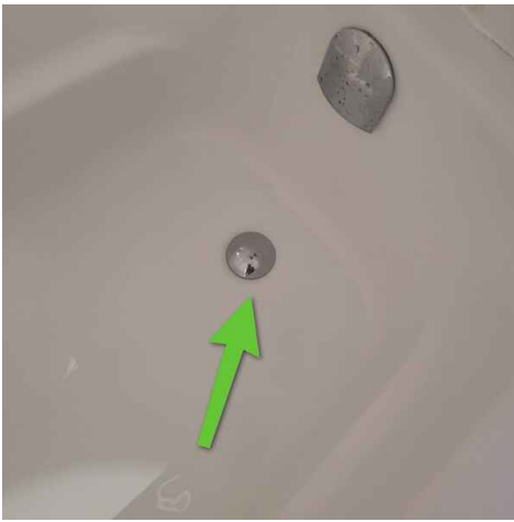
Tub plug doesn't work
